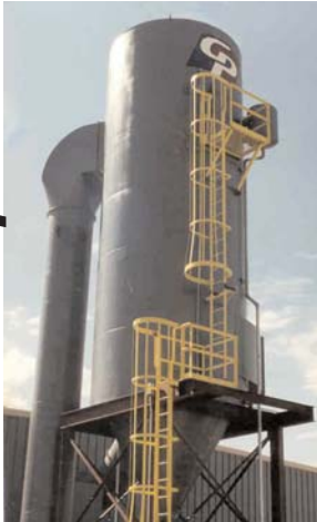
376AC12 Filter handling fibers, epoxy resin from composite fiberglass manufacturing process.
