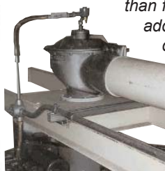
(left) Diaphragm and solenoid assembly.
